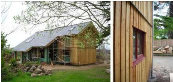
Untreated external cladding; out of contact with the ground and protected overhead by roof.
