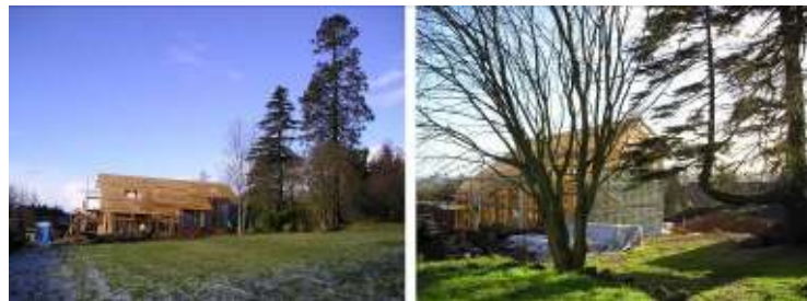
New house under construction in grounds of former country house. Design accommodates and retains mature trees and landscape.
